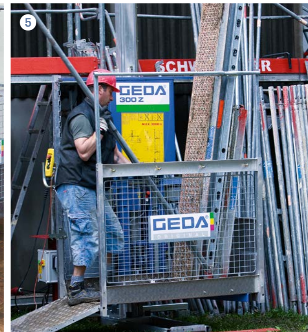
5 Scaffold frame enables safe transport.
