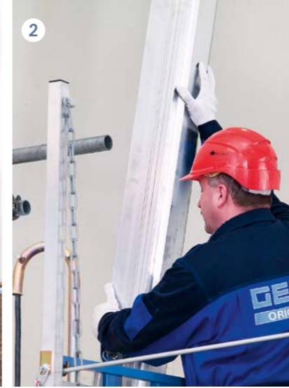
2 Assembly of the aluminium masts by only one person.
