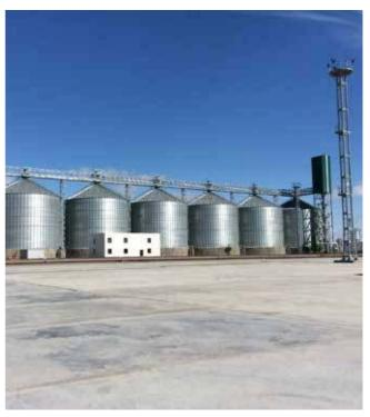
Our silos with a cylindrical body and 30° sloped roof are designed to store grains, seeds and pelletized products.
