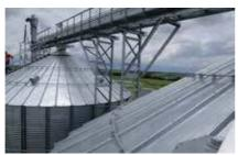
The **lateral support** is bolted to the silo stiffeners. Used for light machinery in silos of up to 24 m in diameter. Additionally, an oblique support can be added to the lateral support depending on the silo and catwalk model.
