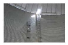
The **inner silo staircase** makes easy access to the silo for maintenance tasks and visual analysis of the product.
