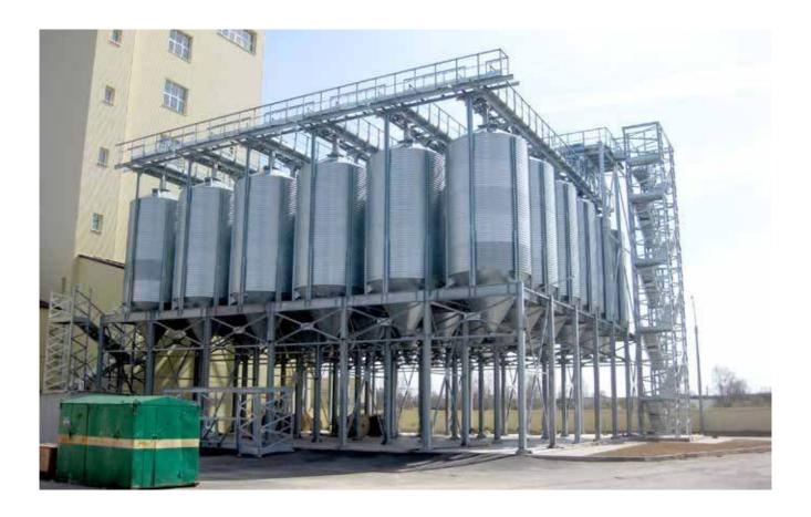
We design and manufacture bulk silos with **support structures** for truck or train drivethru. This structure is made up of rigid bare double-T laminate profiles built in S275JR hot-dip galvanised steel. The standard silo to ground outlet height is 4500 mm with the possibility of adapting to the customer's needs.
