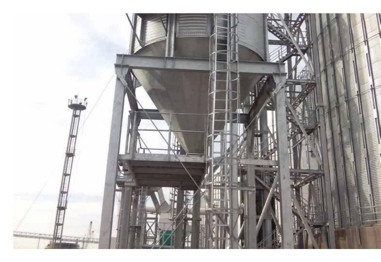
Structure-based truck/train load silos are designed for the storage and later dispatch of bulk products such as granulates, flour, etc.
