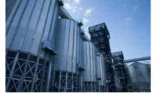
Our range of hopper silos covers capacities ranging from 43 m<sup>3</sup> to 2,016 m<sup>3</sup> with diameters from 3.82 metres to 10.70 metres.
