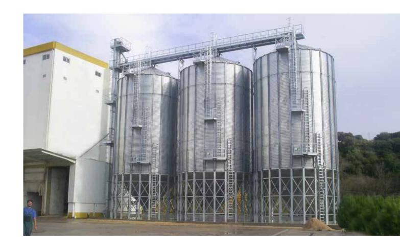
They are designed to store grains, seeds, legumes, pellets and other products that require special storage conditions. The stored product stays off the ground to prevent moisture gaining and lower the possibility of breakage.
