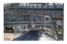
**Cap support** supports the catwalk and is placed above the top cover of the silo roof. There are different types based on the machinery performance and type of catwalk.
