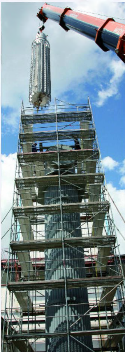
Assembly of CP dryer
