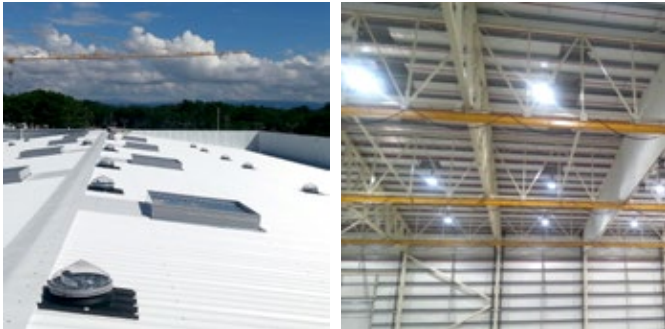
3- Application in ribbed sandwich panel
