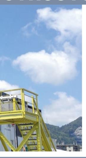
Stairways, walkways and work platforms are built with pultruded profiles, FRP gratings and stainless steel accessories in accordance with EN ISO 14122 standard (Permanent means of access to machinery) within the framework of Directive 2006/42/EC (Machinery Directive).
