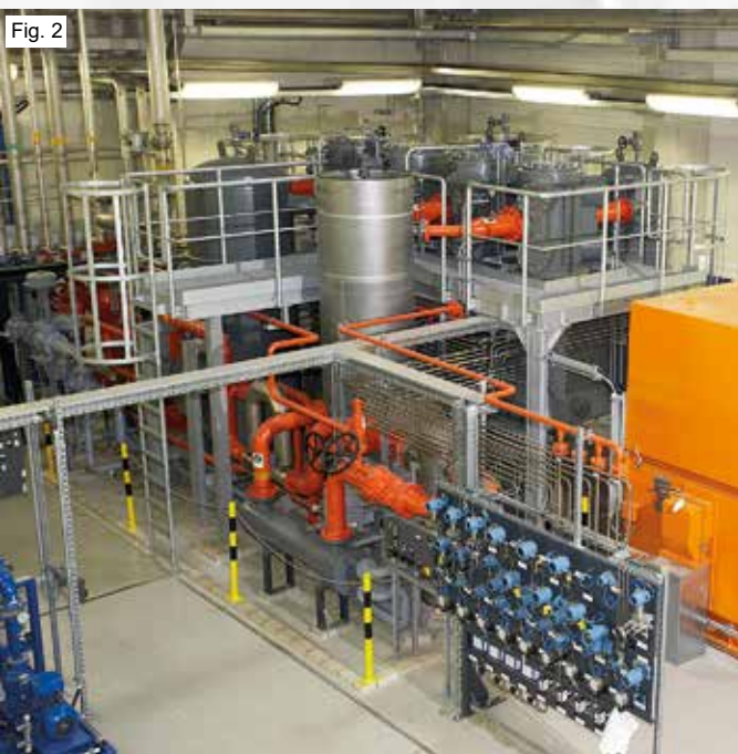
Fig. 1: H 2 import compressor unit, type Bx45, 6 cranks, 43,000 Nm 3 /h
