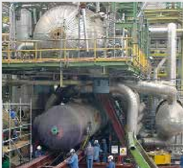
Replacement of a waste heat boilers under BORSIG supervision with mobilization of local personnel
