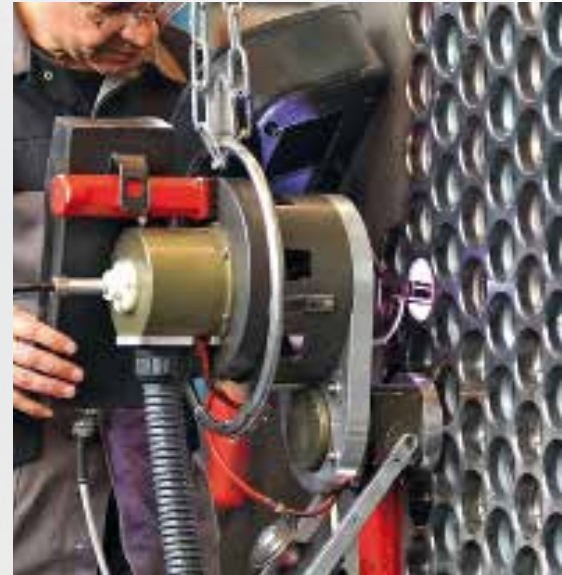
Automatic full penetration tube to tubesheet welding
