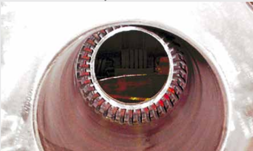
Reinforcement ribs on water side of the gas inlet nozzles
