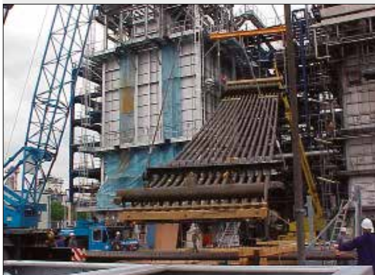
Installation of BLQ
