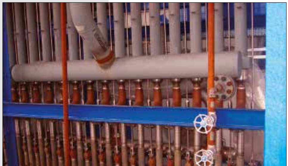
BLQ in the furnace structure
