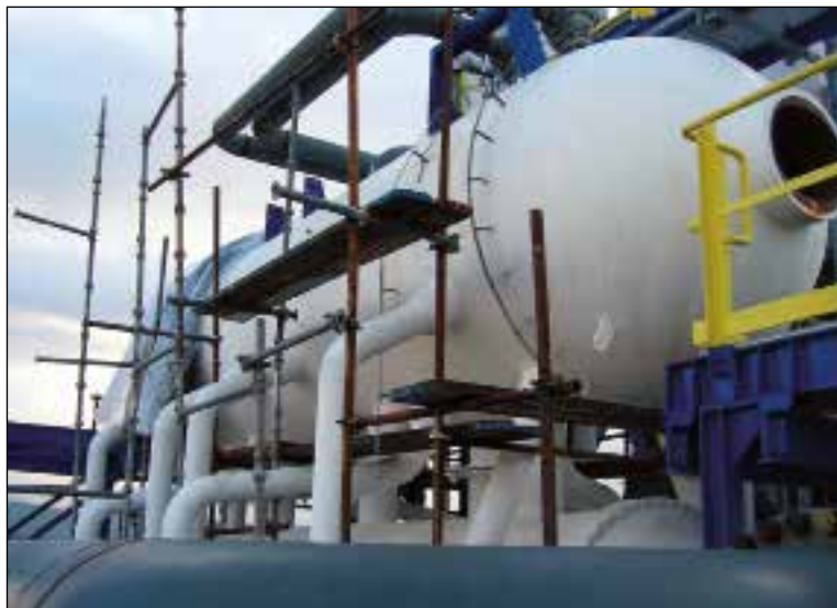
Secondary Transfer Line Exchanger / Steam drum Unit
